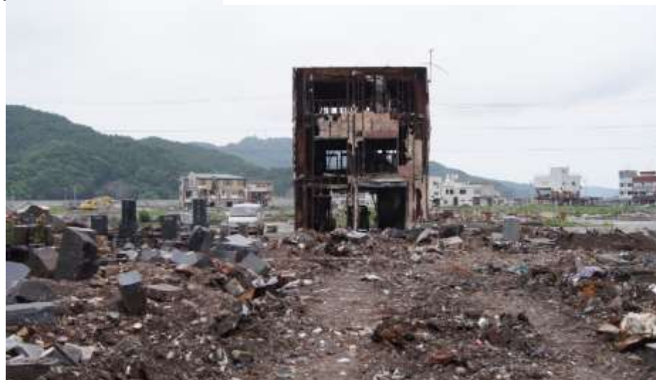
Destroyed steel-made building
