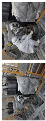
C-主蒸気隔離弁
