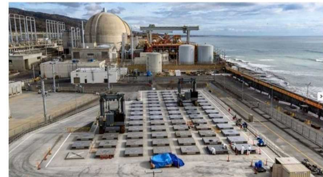
The dry used fuel storage facility at the San Onofre plant in California (Image: Southern California Edison)
