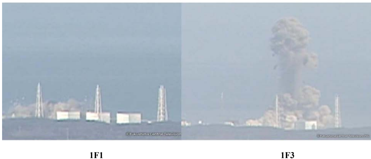
Figure 6-14. Images of 1F1 explosion compared with 1F3 explosion. (Courtesy of FCT [214])
