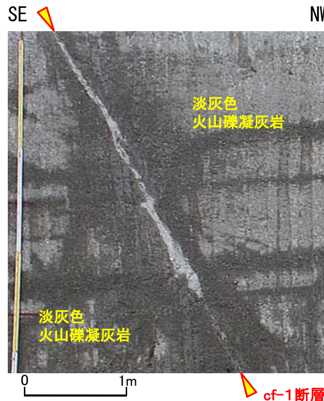
掘削法面①
