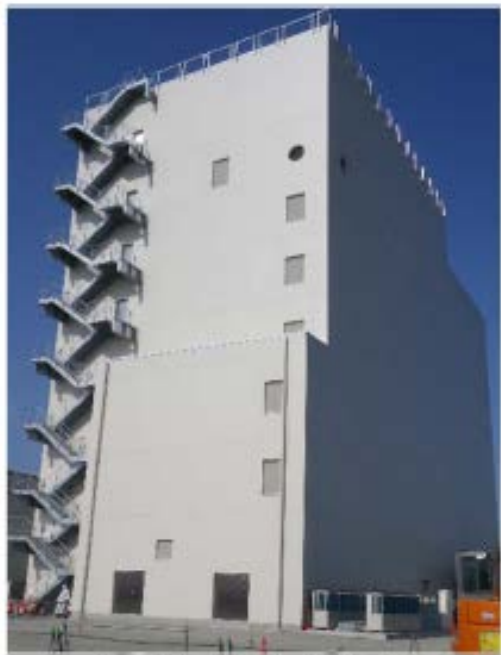
Large Rest House
