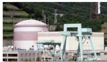
Tsuruga Unit 1 of the Japan Atomic Power Company (Source: the Japan Atomic Power Company)
