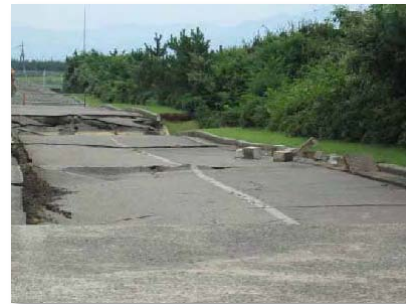
State of the on-site road of the Kashiwazaki Kariwa Nuclear Power Station after the earthquake (Source: TEPCO)
