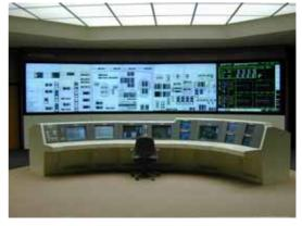
Fig. 12-2 Main Control Panel of the Latest PWR -proto type-
