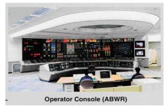
Fig. 12-1 Main Control Panel of ABWR
