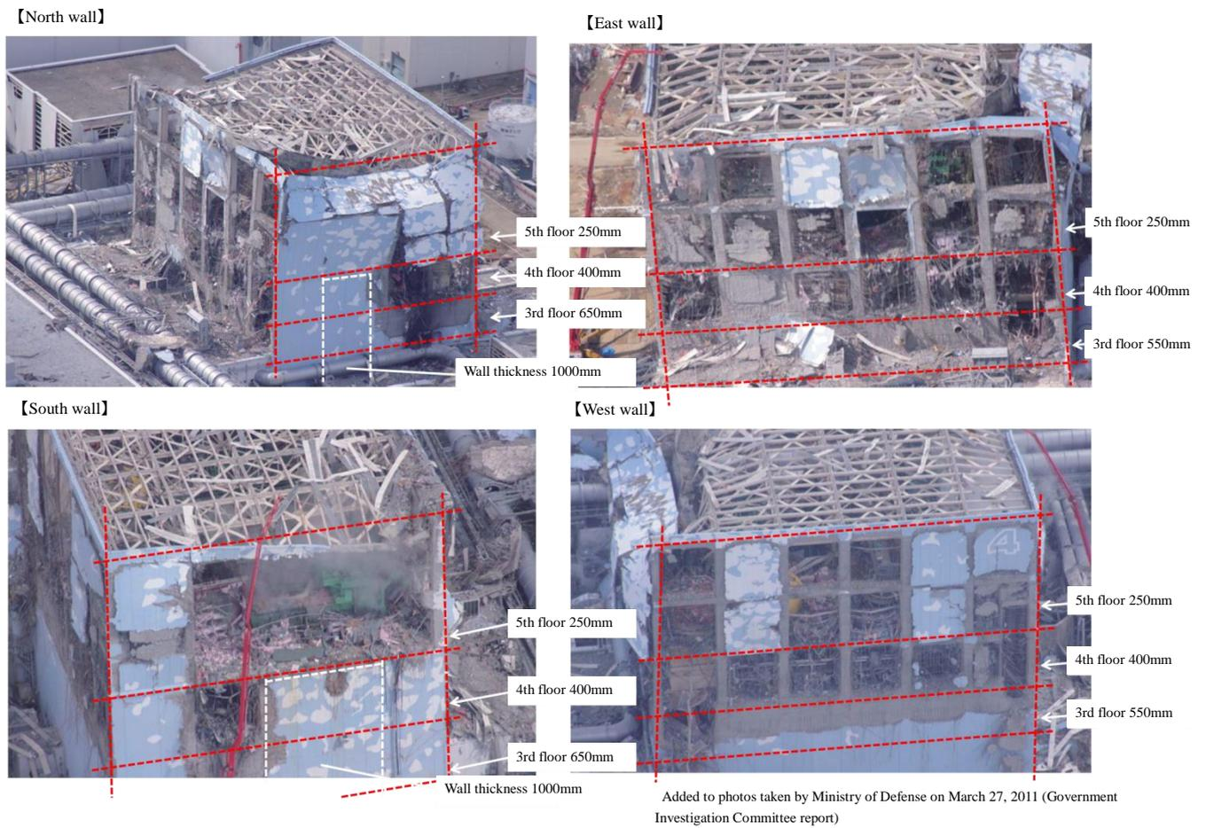
Figure 7.14 Traces of Damages on the Reactor Building (east, west, south, and north walls)
