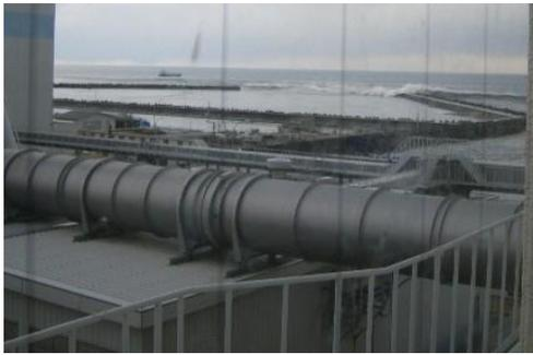
Photo 2 (Tsunami 2-1 flooded the premises (height: O.P.+ 10 m).)
