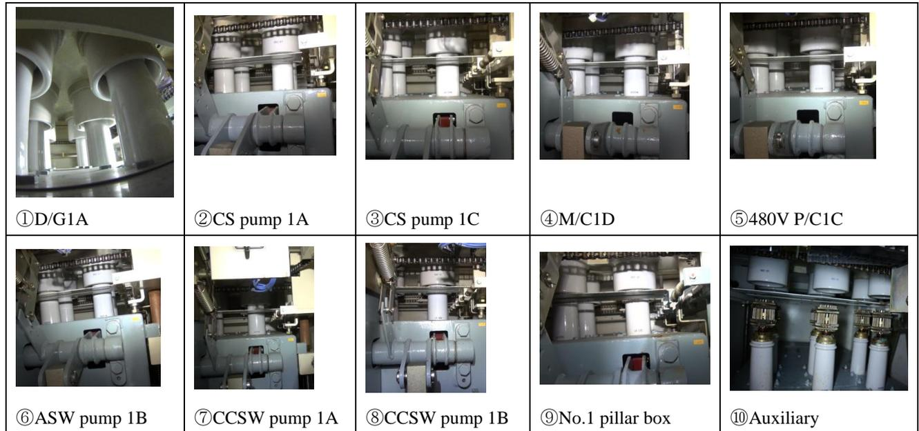
\*Each number indicates a cabinet number and each apparatus name indicates the destination in which the circuit breaker is connected.
